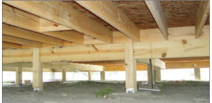
**Simple Foundation** Any foundation can settle, but a raised wood floor system makes leveling or repairs simple.
