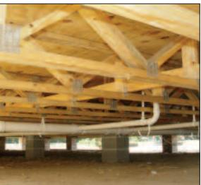
**Soil Variations** – A raised wood floor foundation can be a cost-effective solution to construction in poor soil conditions, where movement of expansive clays or the subsidence of organic soils is a concern.
